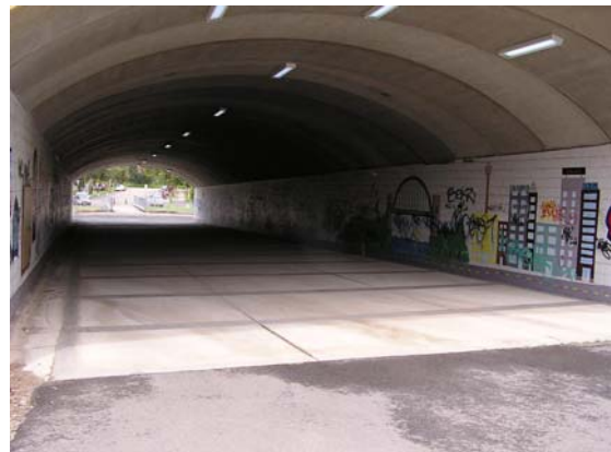
Arinya Street underpass
