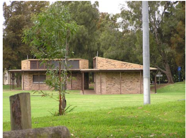
Beaman Park pavilion
