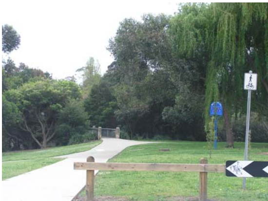
Footbridge over Cooks River at Karool Avenue
